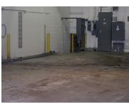
Drain area eaten away- 2<sup>nd</sup> Drain also destroyed- General Floor area deeply etched Repair Procedure:
