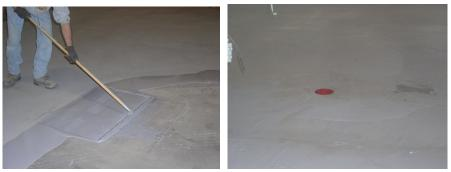
Application of ShurBond 550 coating to surface. Details of newly finished drain.
