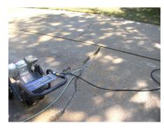
Cracks prepared by grinding and power washing.
