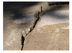
Cracked slabs brought up to level and repaired with ShurBond 550 Epoxy Adhesive and ShurBond 100 Polymer Concrete. Picture on the right also shows severly spalled area
