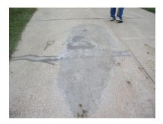
Single coat of WOHL Concrete Coating (low film build for better results use two coats or WOHL Concrete Surfacer)
