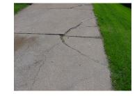
Cracked slabs brought up to level and repaired with ShurBond 550 Epoxy Adhesive and ShurBond 100 Polymer Concrete and the Finished coated with Wohl Surface Coating.
