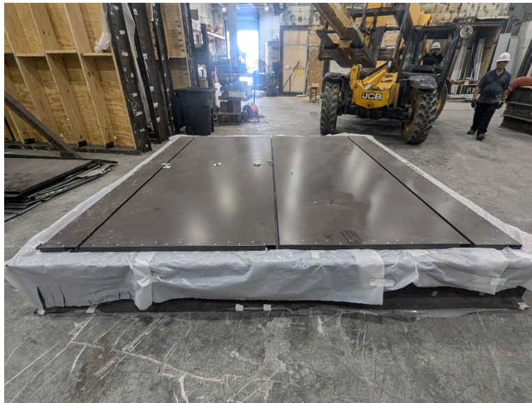
Photo No. 2 Installed Panels – End View
