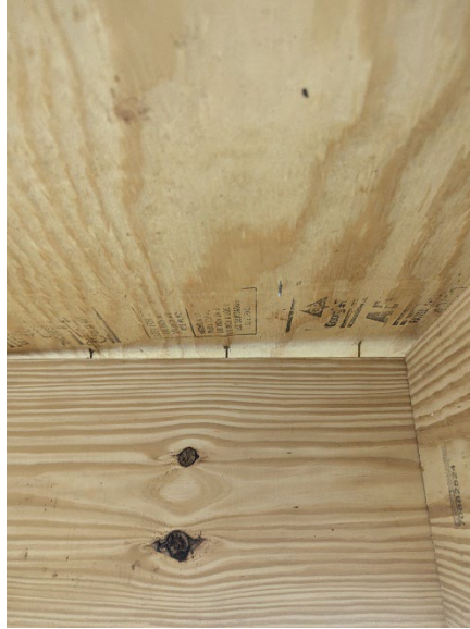
Photo No. 4 Plywood Failure – Specimen #3
