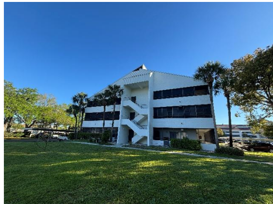
Picture 4: Typical South Elevation
