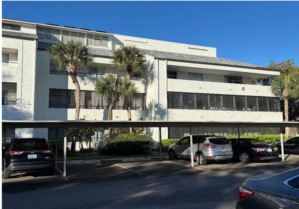
Figure 9: Typical East Elevation – Building 4 (No visible structural distress observed)
