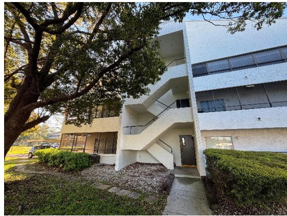
Picture 2: Typical North Elevation
