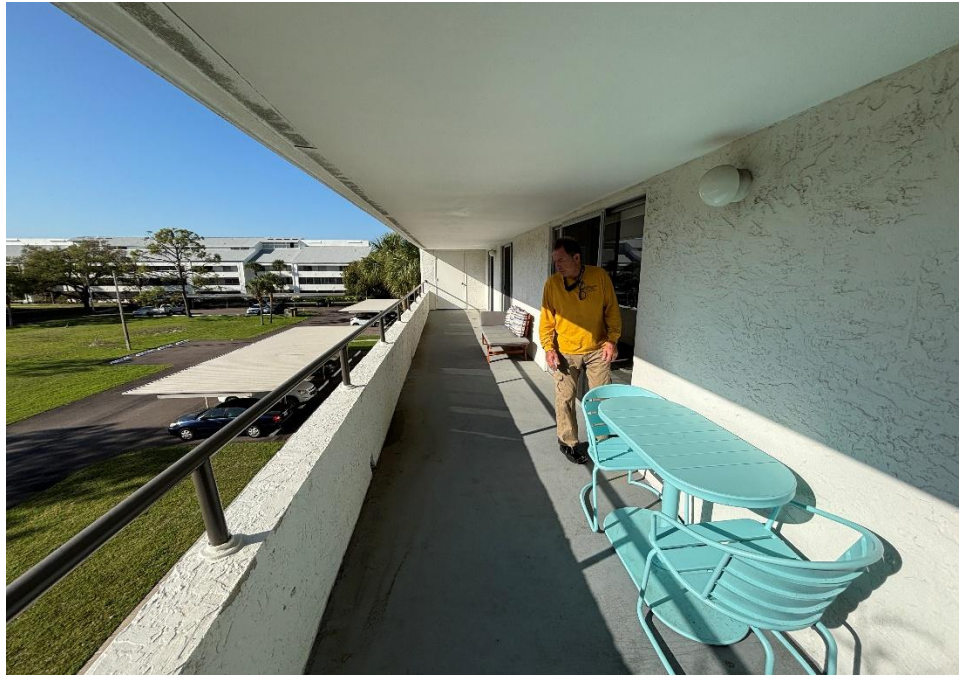
Figure 5: Typical balcony condition showing no visible signs of structural distress – Building 2.
