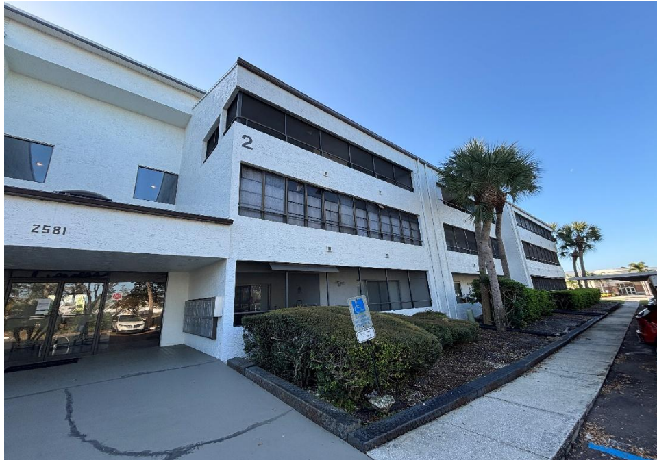
Figure 1: Typical West Elevation – Building 2 (No visible structural distress observed)
