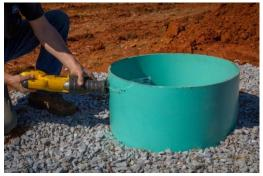
**Step 11:** Harco Fittings LLC drain basin top is easily adjusted with saws-all to adjust height of the grate or cover to final grade elevation. Riser sections are available to raise final elevation as well.
