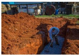
**Step 2:** Ensure bedding is leveled and compacted to support drain basin and pipes.
