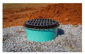
**Step 12:** For ALL vehicle / traffic load applications, pour a concrete collar under and around the ductile iron grate frame per project engineer or Harco Fittings LLC recommendations.
