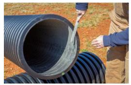
**Step 5:** Remove burrs from cut end of pipe. Clean first two pipe corrugations. Use only Harco Fittings LLC supplied pipe gaskets – zip-tied to each drain basin.
