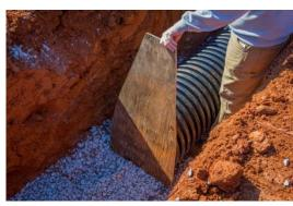
**Step 8:** Place board or pipe installation stub over end of pipe to protect pipe during install.
