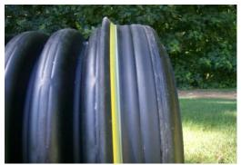
**Step 7:** 12" and larger pipe gaskets straddle first two corrugations, color on gasket toward end of pipe, fin on gasket sitting over second corrugation. Clean area then lube gasket <u>AND</u> inside basin bell. (Pipe lube supplied by distributor or pipe company)
