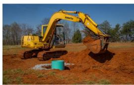
**Step 10:** Knife backfill material under and around pipe and drain basin outlets. Place approved backfill material in lifts and compact following ASTM D2321 plastic pipe installation guidelines.
