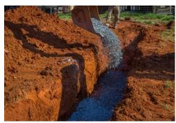
**Step 1:** Excavate trench to width and depth required for pipes being installed. Use ASTM D2321 guidelines for bedding and backfill material and compaction requirements.
