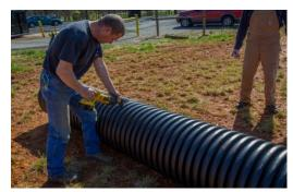
**Step 4:** For corrugated polyethylene pipes, remove bell or spigot so full size corrugations will hold gasket and install into drain basin bell. Cut pipe in valley between corrugations.
