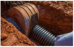
**Step 9:** Gently push pipe into drain basin bell with hoe bucket or use spud bar. Re-level basin.
