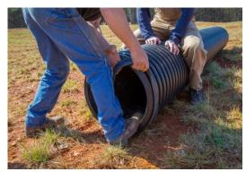
**Step 6:** Install pipe gasket to straddle between first and second pipe corrugations. Start at bottom and work around to top.
