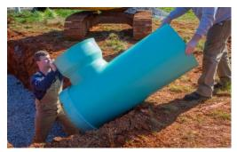
**Step 3:** Lower drain basin into trench, set in place, and level prior to pipe installation. Place backfill so basin is stable during pipe install.
