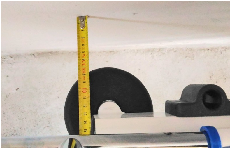
Recommended positioning from rear wall at least 8cm from the corner roller buffer
