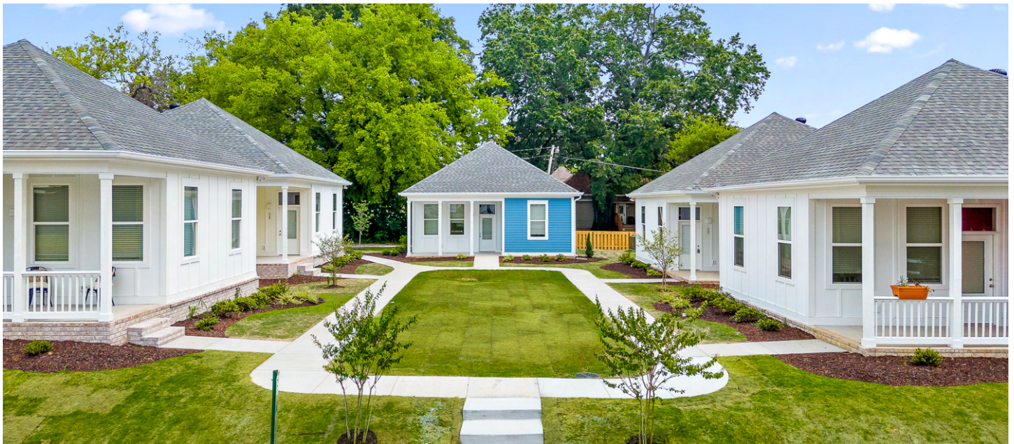
Finished Cottage Court on Vance Ave
