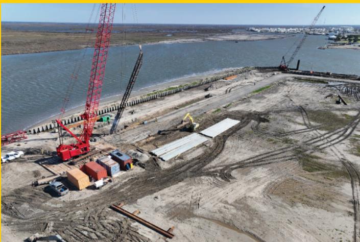
SLIP D BULKHEAD CONSTRUCTION
