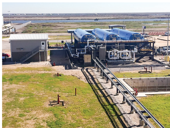
Fig. 3. The three tanks at Harvey Gulf International Marine's bunkering facility in Port Fourchon are capable of holding 90,000 gal of LNG each.
