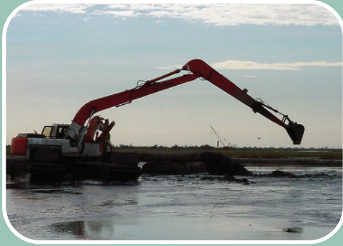
Dredge pumping and shaping of material in the Maritime Forest Ridge
