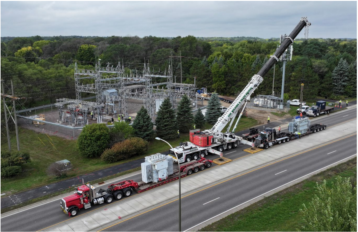
The old transformer is on the red truck; the new transformer is on the black truck.
