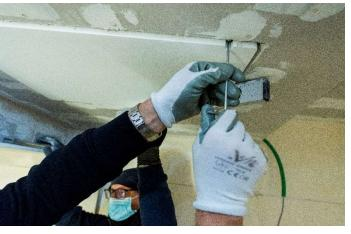
7 Check each corner and on both axis. **IMPORTANT**: the loudspeaker surface must be level with the finished wall/ceiling
