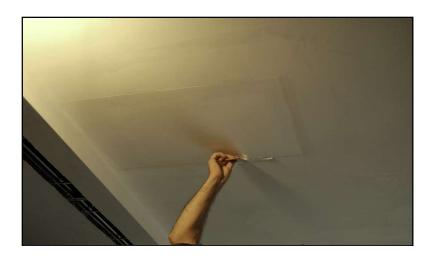
14 Once completely dry, sand and smooth edges. Examine the surface with the work-light and smooth any imperfections.
