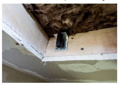
$\frac{\text{NOTE}}{\text{NOTE}}: \text{rubber standoff will compress allowing the loudspeaker to be levelled with walls/ceiling thickness ranging from $1/2$" to $5/8$". Any installation with surface materials other than specified will require different length screws, alterations to the standoffs and may impede proper installation of the loudspeaker.}$
