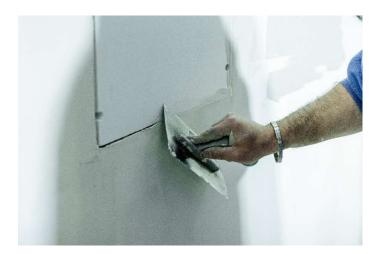
NOTE: If the compound falls inside the cavity, add joint compound to thicken the mix. Time may vary depending on the temperature/humidity on the room.
