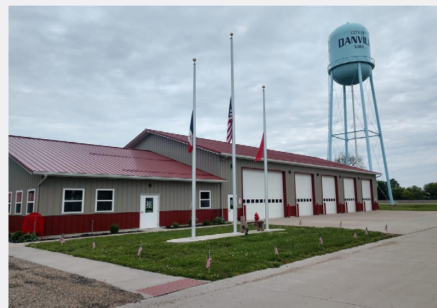
The new Danville Fire Station, completed in 2019
