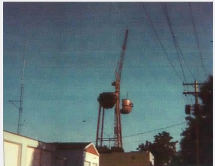
The new water tower, under construction in the late 1980s
