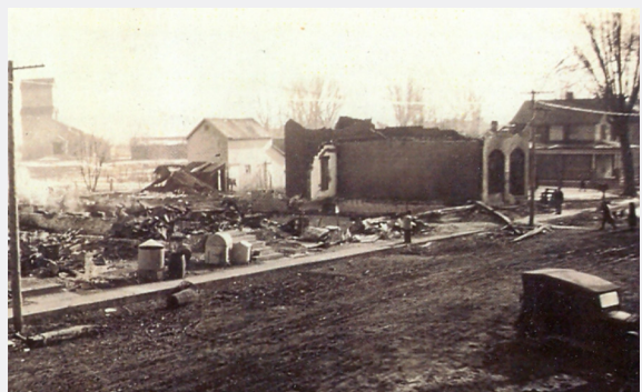
The aftermath of the fire on January 24, 1921, showing the east side of Main Street downtown
