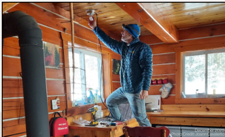
Dave Fanslow installing solar light over kitchen counter.
