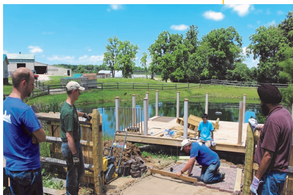
New pond deck being built by GE volunteers
