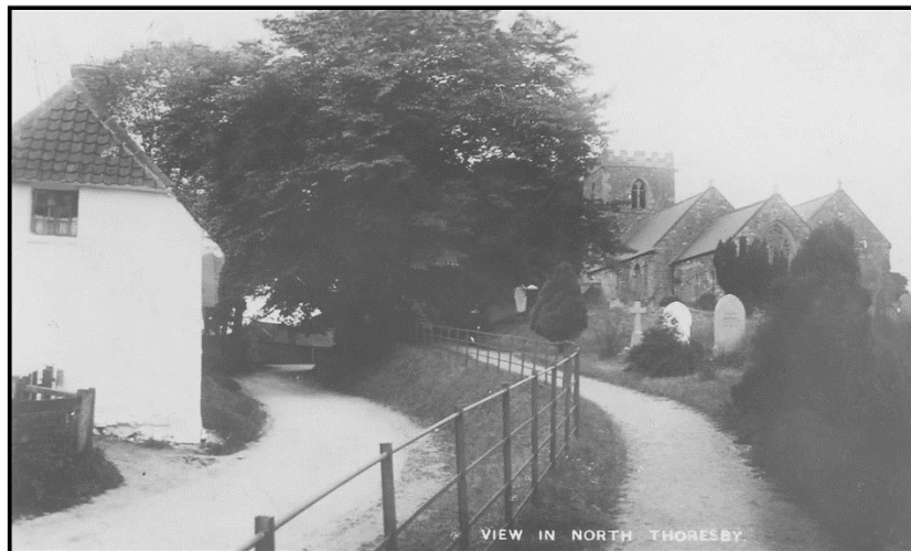
Jubilee Cottages - note the sunken road. Church Farm buildings in the background.
