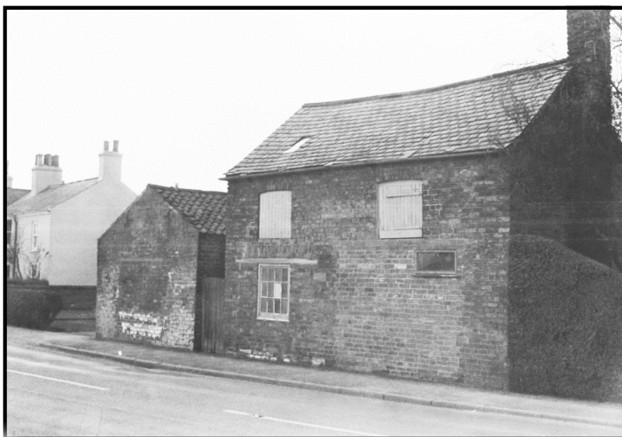
The Saddlery before conversion.
