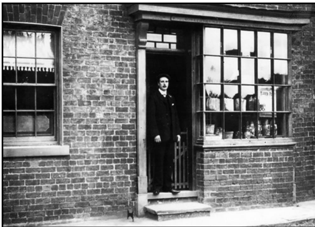
Note the brick bonding scheme - three 'stretchers' between a header
