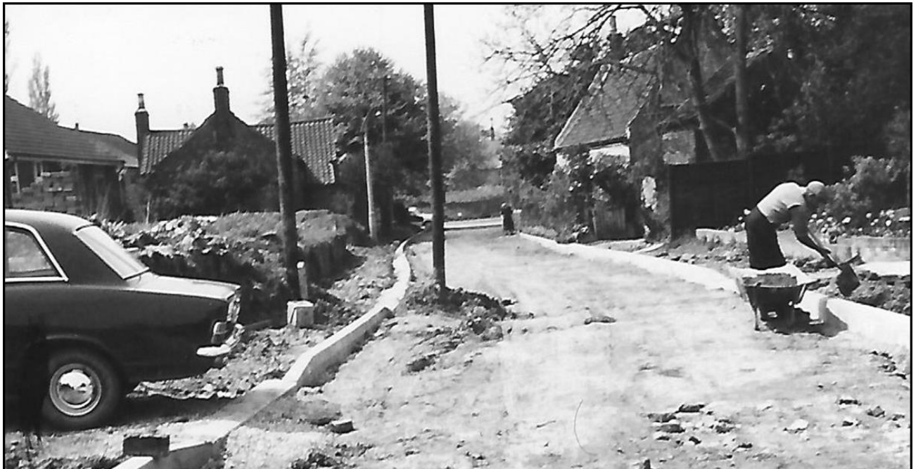
Haith's Lane, 1964. Old brick built cottage to the right and the old St Helen's Schoolroom to the left - both demolished during development.
