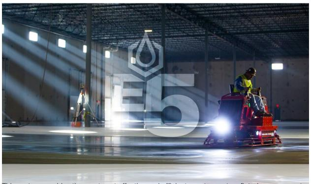
This system provides the most cost effective and efficient way to create a flat, dense, concrete slab for polishing. Please refer to Manufacturer Technical Data Sheets and refer to this system guide for details of the system implementation key QA inspection steps.
