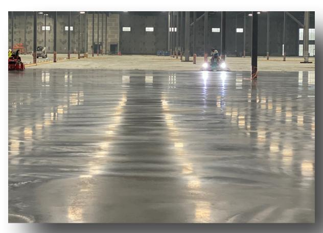
requirements of making a most consistent "canvas" to be polished. This step is even more critical than the polishing step to produce a consistent outcome.
