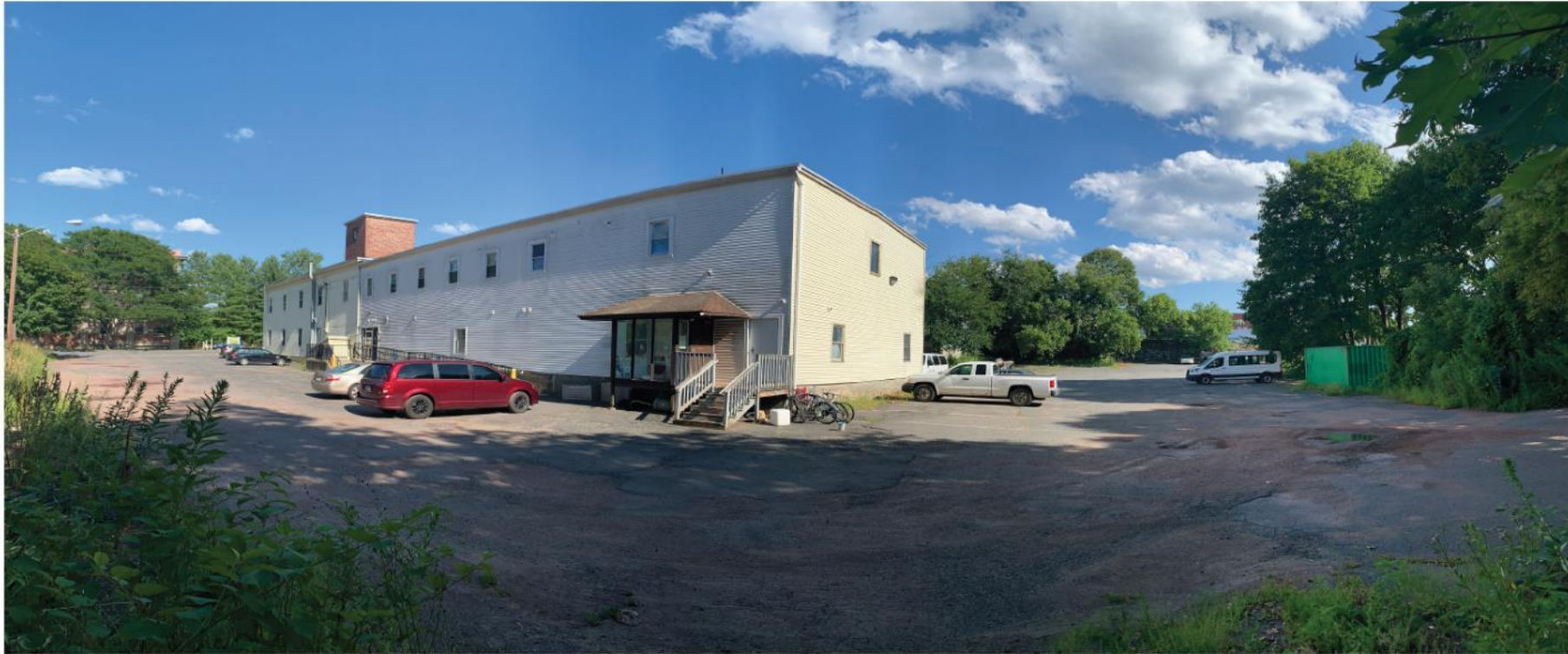
EXISTING VIEW OF NORTH FACADE LOOKING SOUTHEAST
