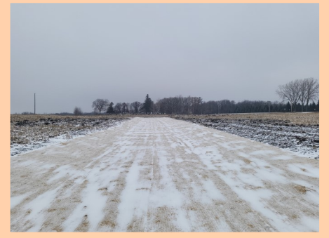
Completed grassed waterway with erosion control blanket.
