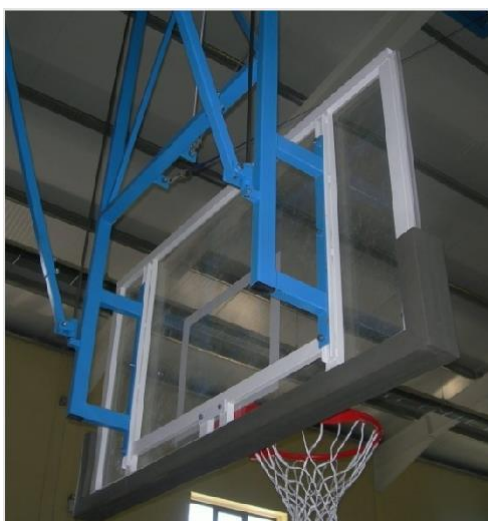
Fig. 2 Drop down goal support structure example
