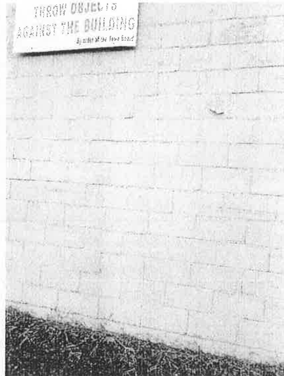
Paint Stripping & Mortar Damage
