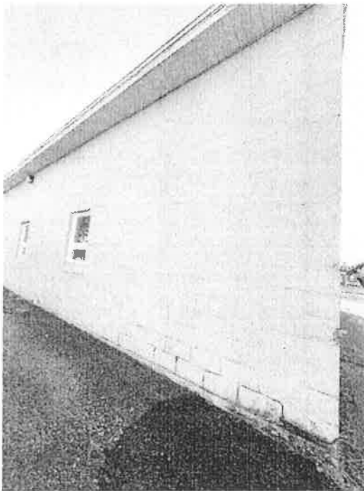
Damage From Water Infiltration
