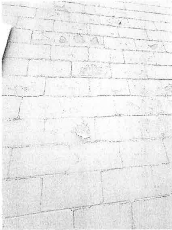
Paint Stripping & Mortar Damage
