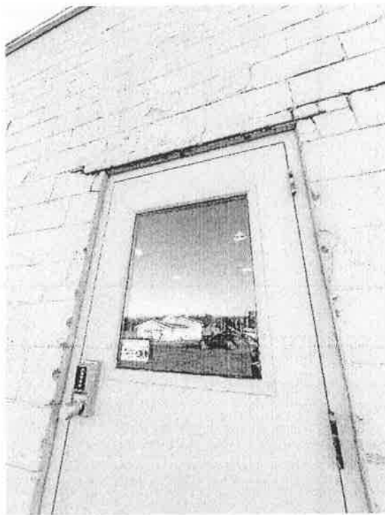
Man Door In Need of Replacement
