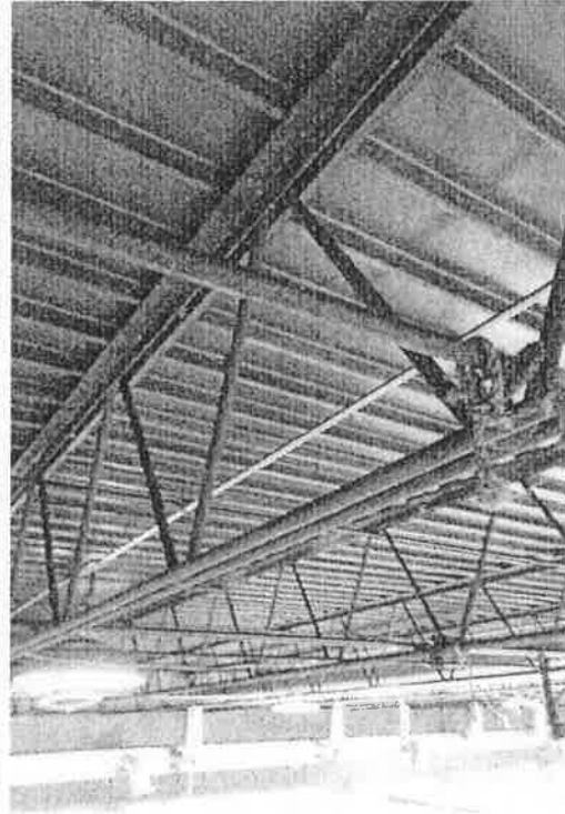
Bar Joists & Composite Deck
