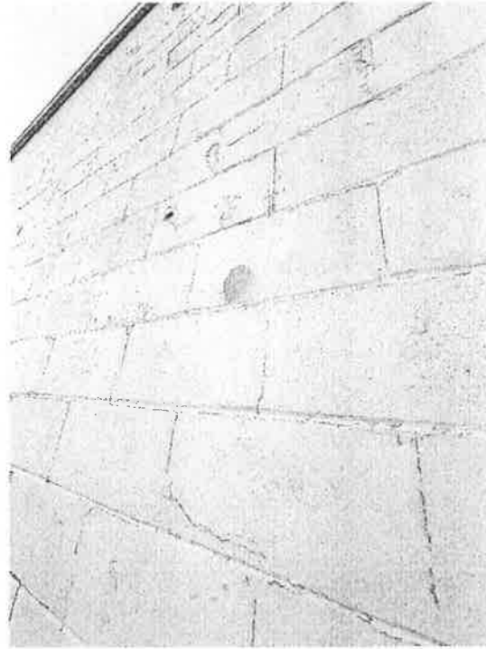
Paint Stripping & Mortar Damage
