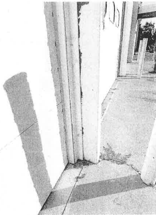
Paint Flaking & Weather Enclosure Deterioration
