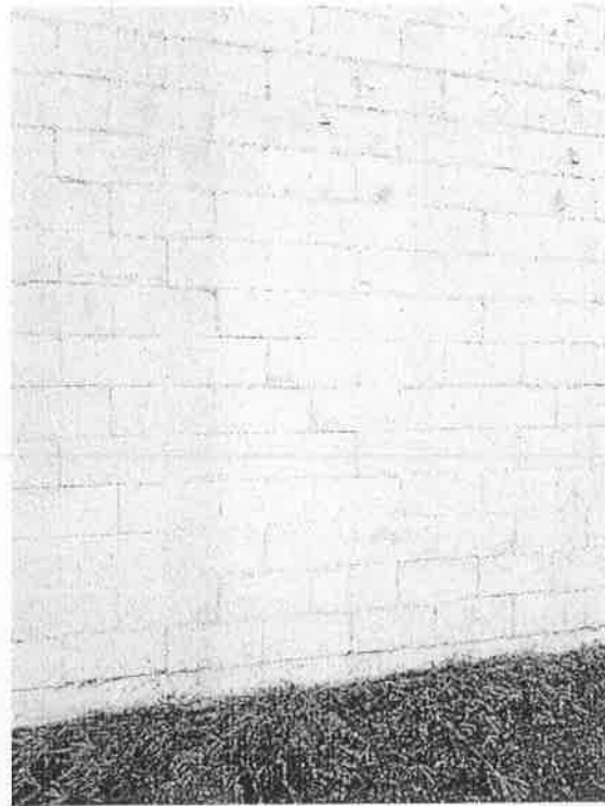
Paint Stripping & Mortar Damage
