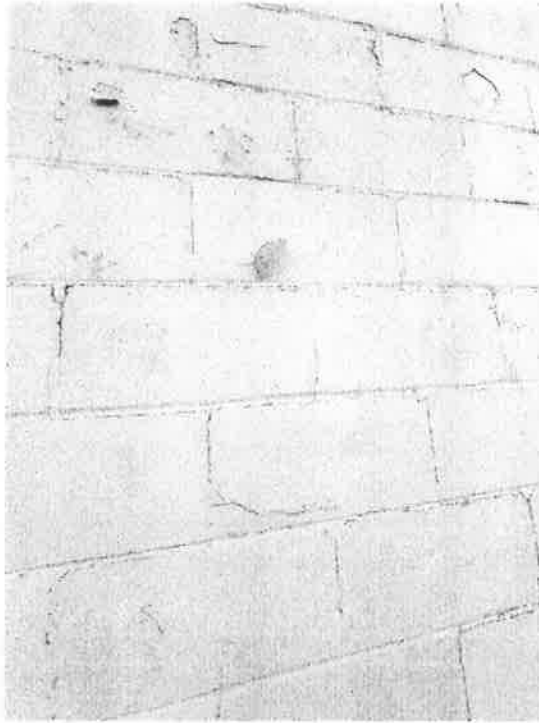
Paint Stripping & Mortar Damage
