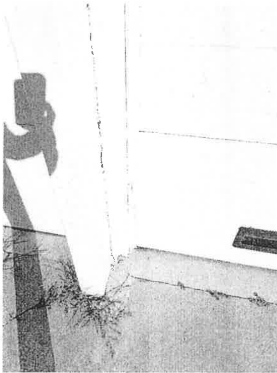
Paint Flaking & Weather Enclosure Deterioration
