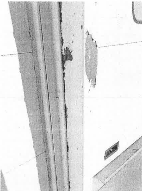
Paint Flaking & Weather Enclosure Deterioration
