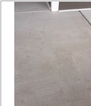
Shrinkage crack
