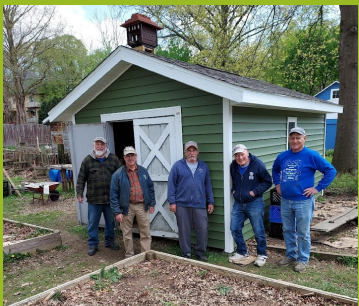
Habitat Volunteers updated the shed on the Buckeye street garden by applying new siding.
