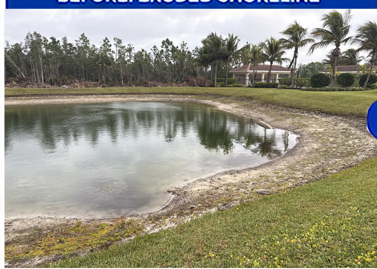
BEFORE: ERODED SHORELINE
