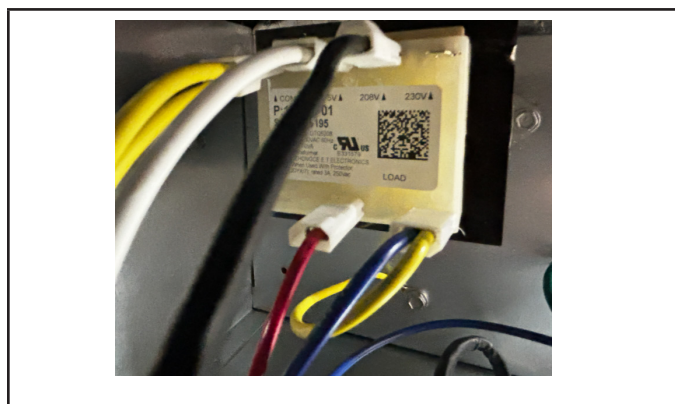
FIGURE 24. Converting Unit from 230VAC to 208VAC
