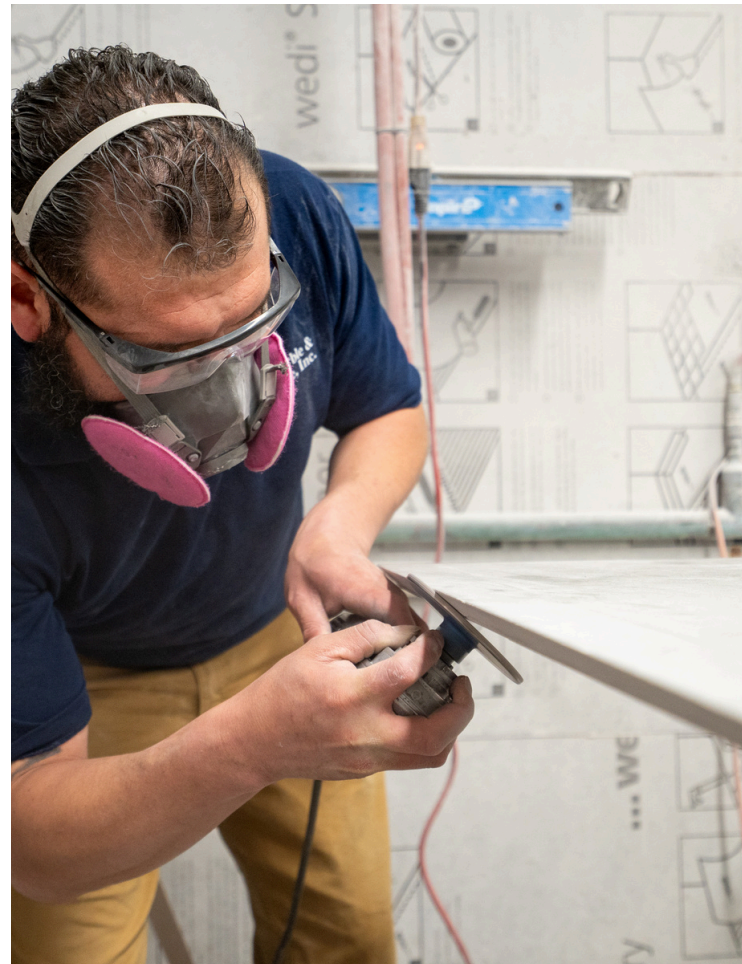
SLAB FABRICATION & INSTALLATION
