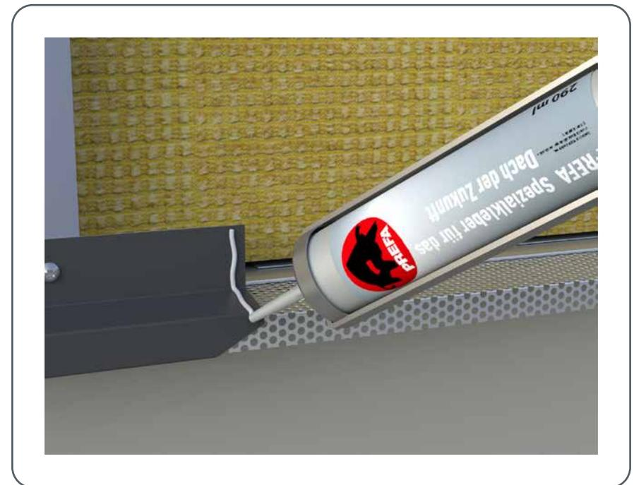
Figure 68 • Drip edge joint
