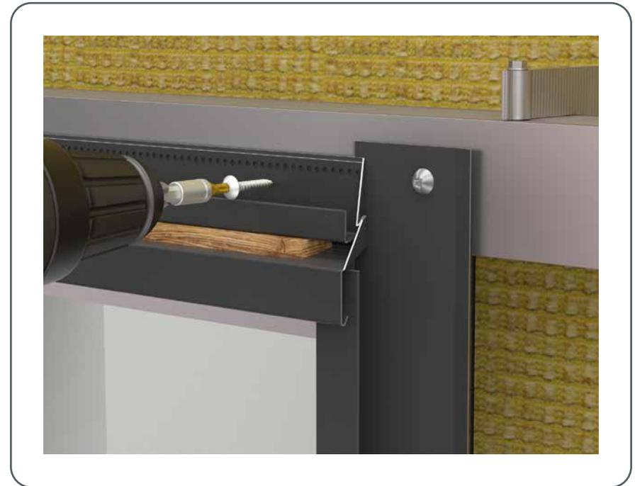
Figure 102 • Installation of perforated profile
