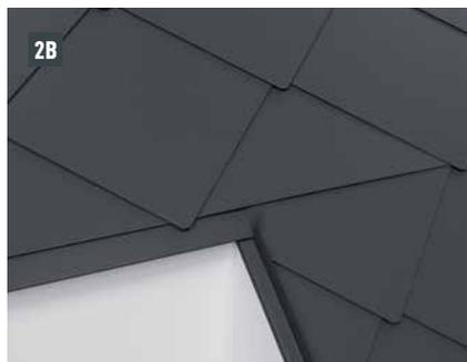
The following row of rhomboid roof tiles can then be installed over the entire width (Image 2A + 2B).
