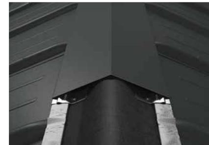
Figure 73 - Ridgedetail with simple ridge cap
