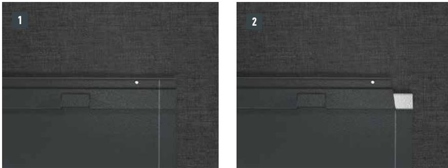
Notch the upper patent fold in the area of the raised edge so that a hook fold remains and bend the R.16 roof tile or the FX.12 roof panel upwards 30 mm at a right angle to the roof surface (Image 1 + 2).
