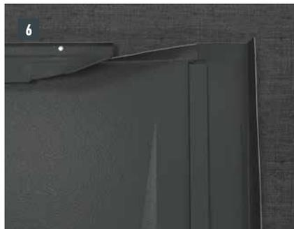
When edging backpart, the upper hook-on seam of the R.16 roof tiles or FX.12 roof panels to be covered is cut at approx. 200 mm and notched. The hook-on seam is bent backwards and the side overhang is bent up 90°. The back part of the surroundings to be installed.
