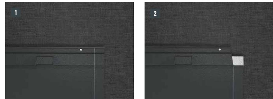
Notch the upper patent fold in the area of the raised edge so that a hook fold remains and bend the R.16 roof tile or the FX.12 roof panel upwards 30 mm at a right angle to the roof surface.
