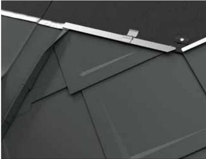
Figure 109 • Roof window surroundings - Special feature of 29×29 and 44×44 rhomboid roof tile
