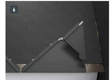
The sloping patent fold is to be notched at the top in the area of the raised edge corresponding to Image 6.
