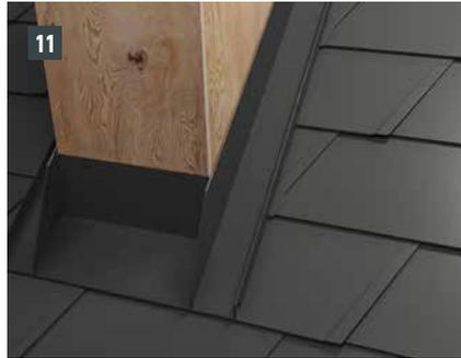
Prepare the surroundings (back and side part) and fix these to the side parts of the substructure with return clips.
