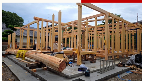
Foundation and frame of the second Kyoto machiya .
