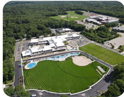
Turf & Athletic Field Installation
