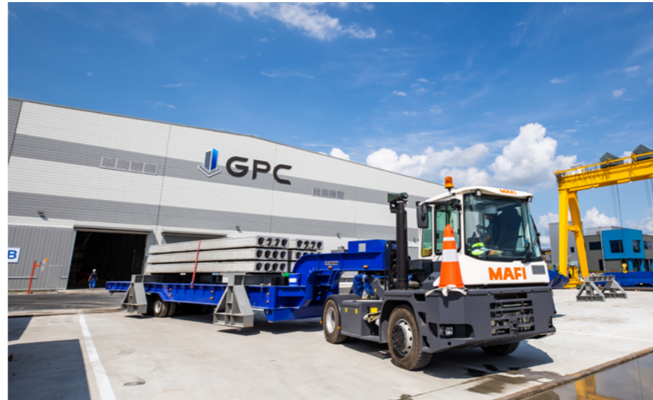
Precast Concrete (PC) plant in Eumseong-gun, Chungcheongbuk-do
