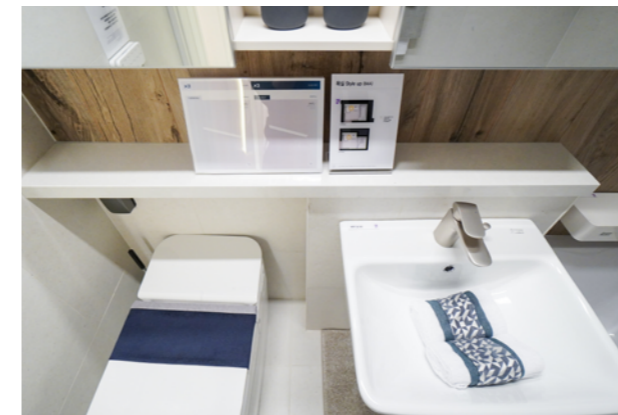
Bathroom Shelf Constructed with Engineered Stone
