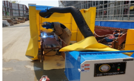
Installation of Portable Screen and Dust Collectors
