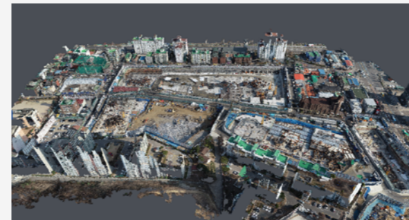
Check the on-site deployment using a drone
