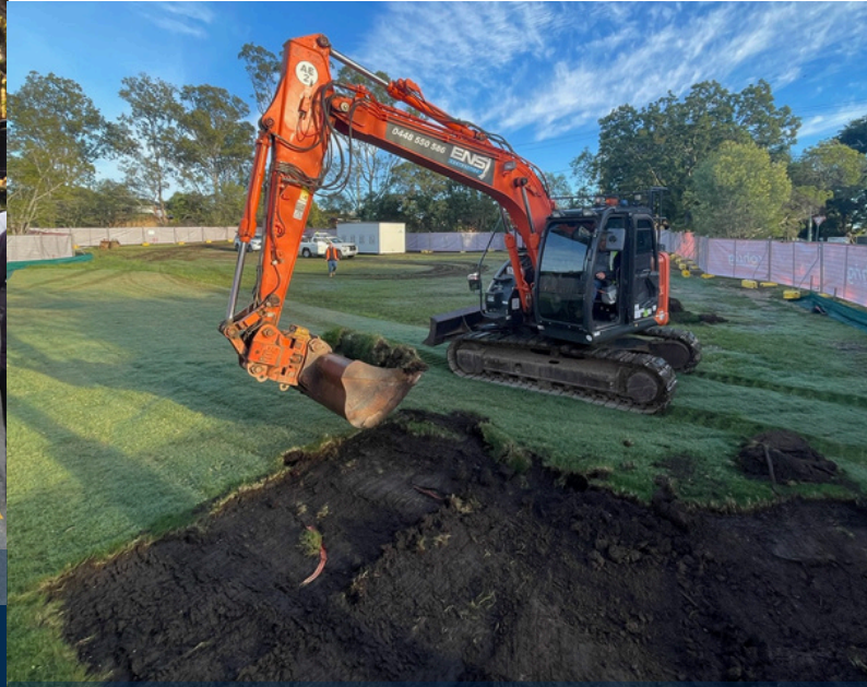
Breaking ground on Stage Two
