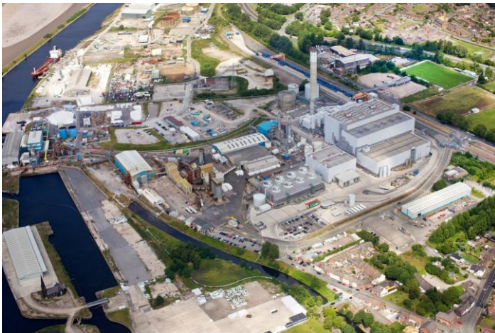
Viridor Runcorn ERF, the UK's largest Energy Recovery Facility
