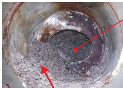
LOAD OF SCALE AT THE OPEN HAND HOLE ON A TUBELESS BOILER
