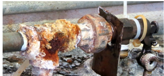
LOOSE COMPOUND FEED TUBE SPILLING COMPOUND OVER THE TOP OF RETURN TANK CORRODING METAL
