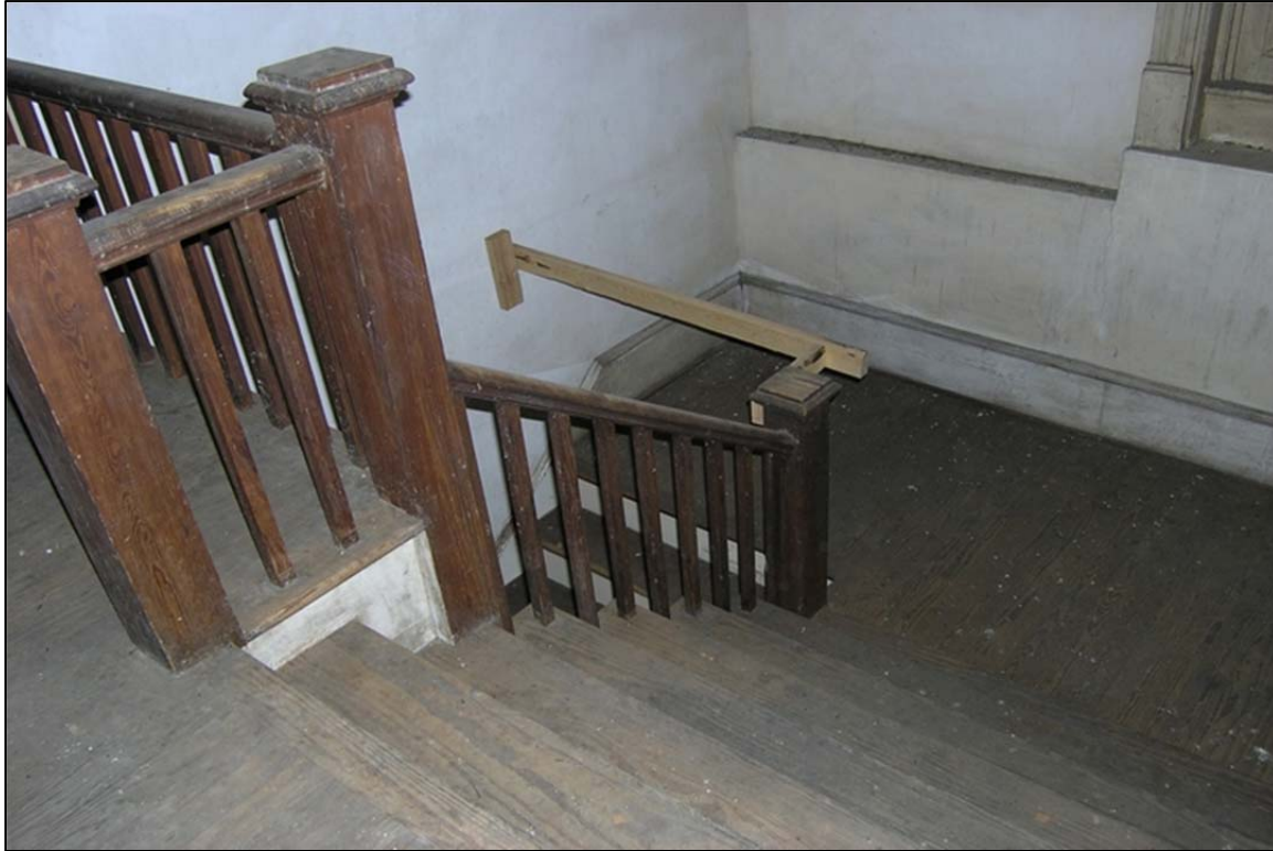
Figure 27. Second story stair rails and landing.
