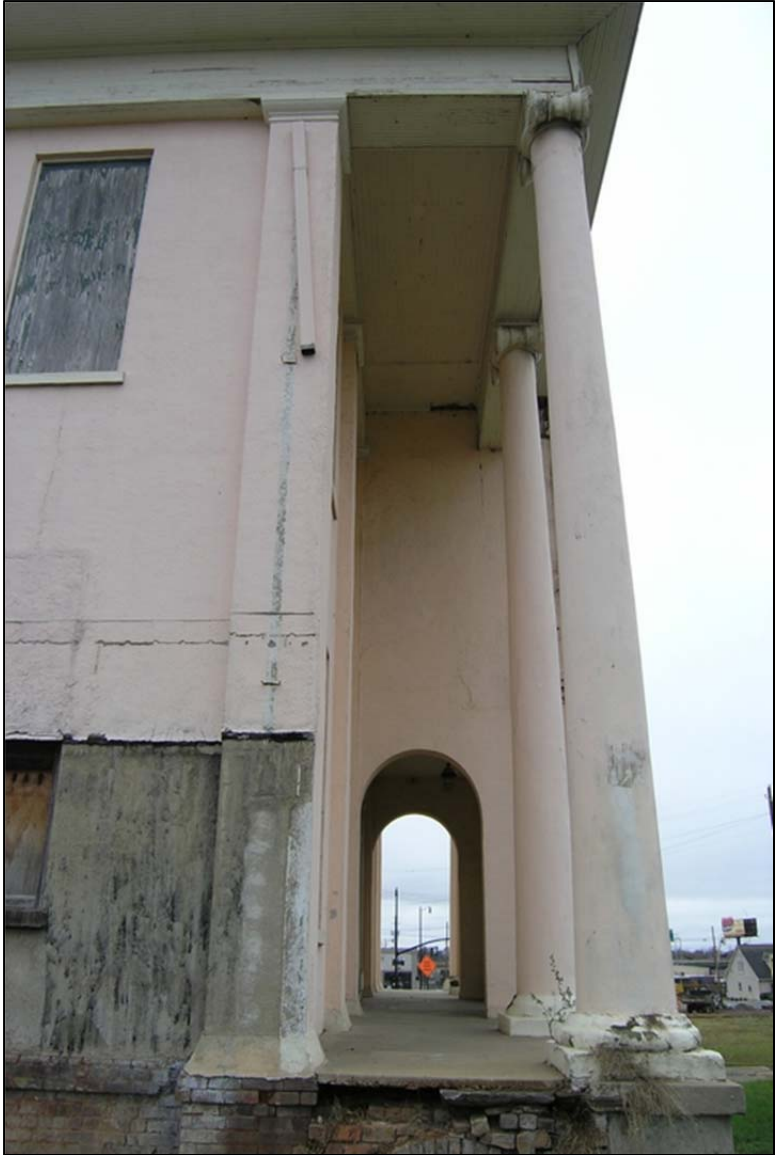
Figure 14. East side of north portico looking west.
