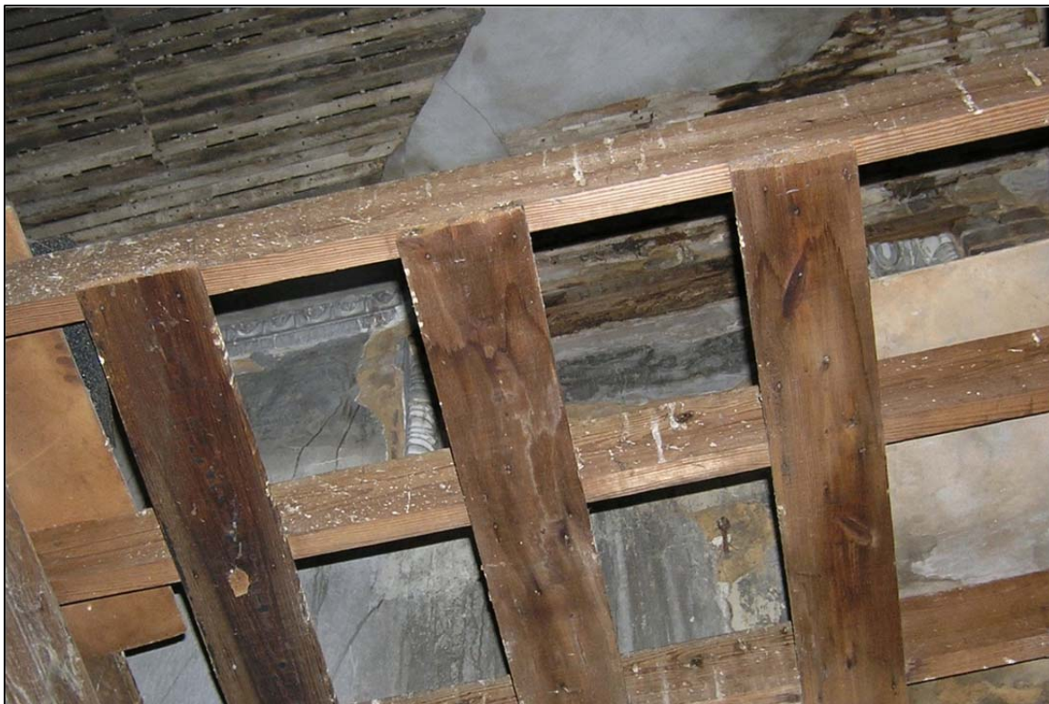
Figure 24. View of original decorative details through frame work of former drop ceiling in tower.
