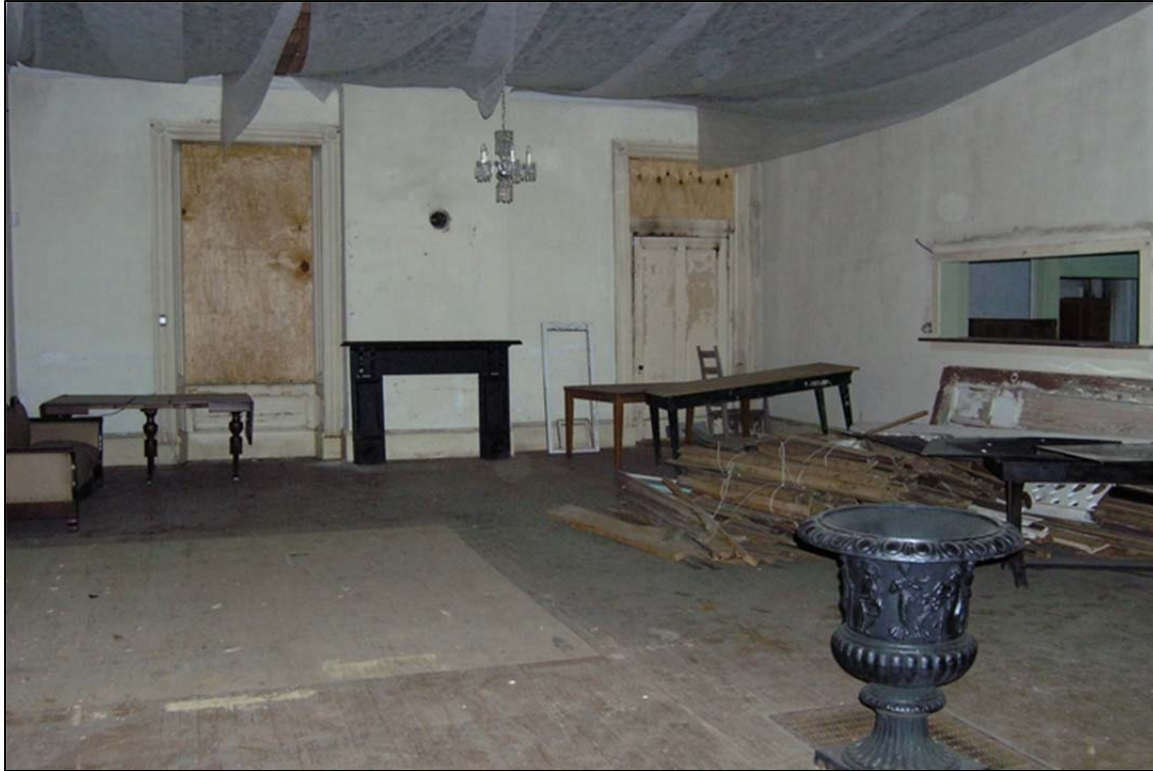
Figure 21. Auditorium looking at the west side of the room.
