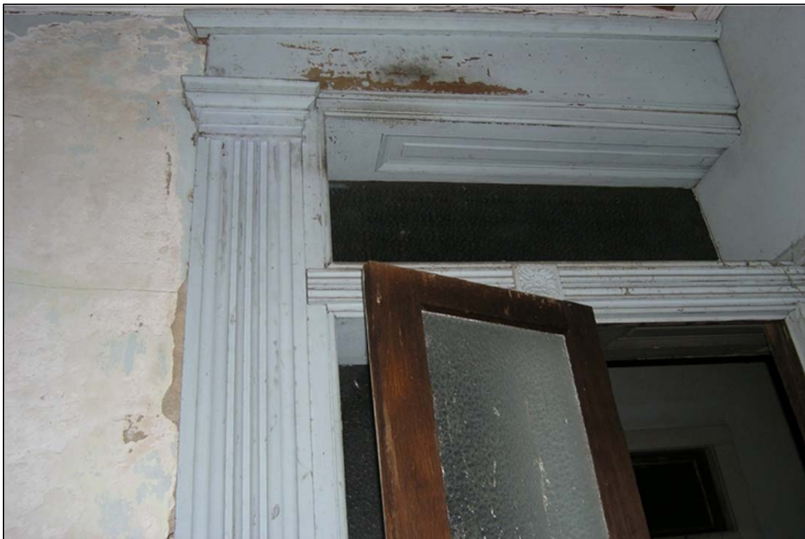
Figure 26. Second story north side frontispiece in tower.
