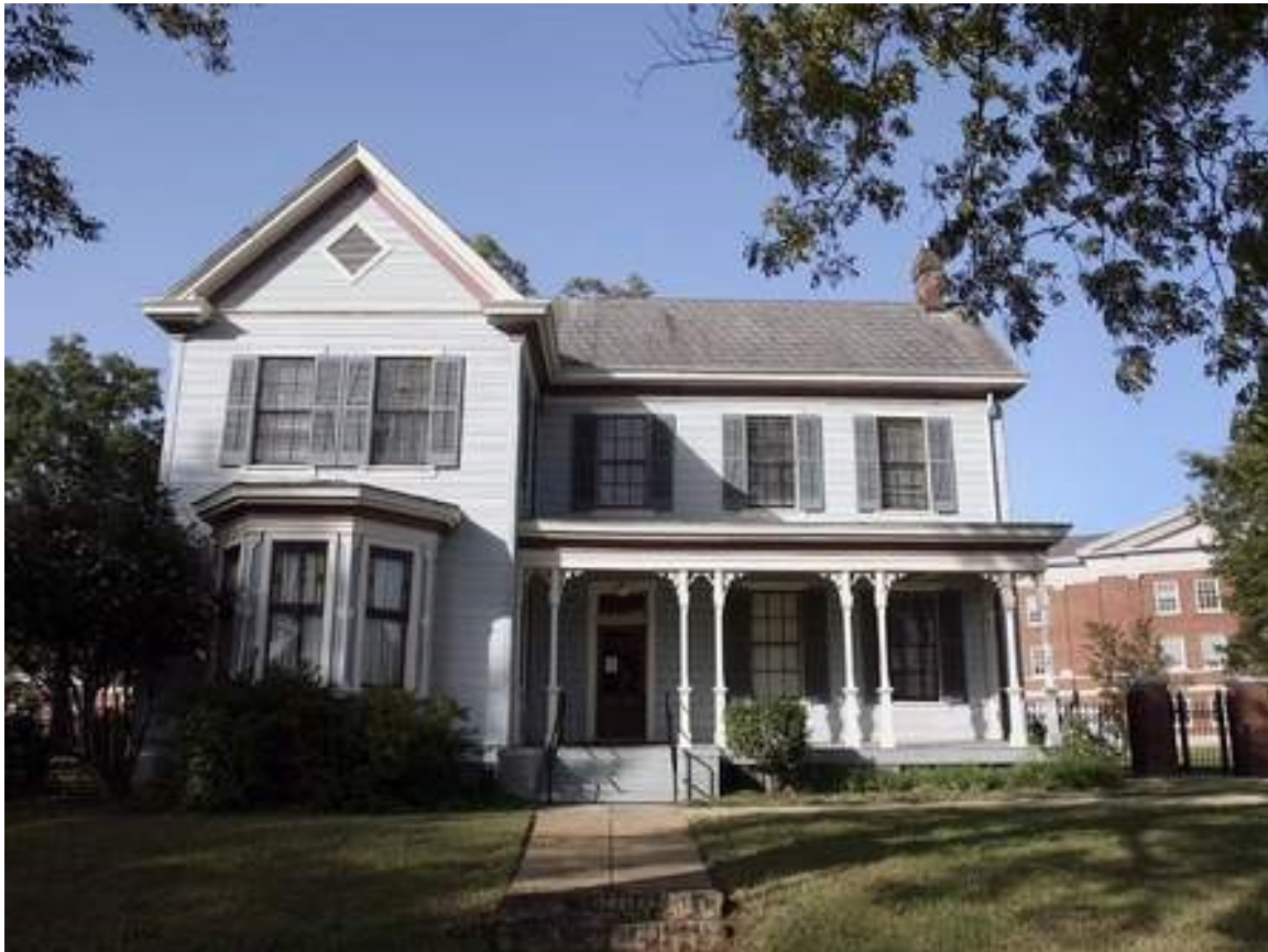
Modern Photograph Before Demolition
