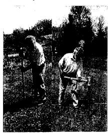
Make a pilot hole for the sleeve and then drive the sleeve half way into the ground with the driving cap.
