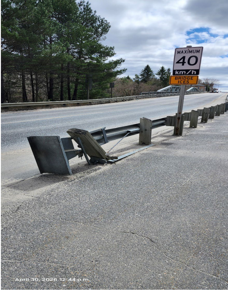
Fig 1. Pictures End Treatment "A" Ontario Street
