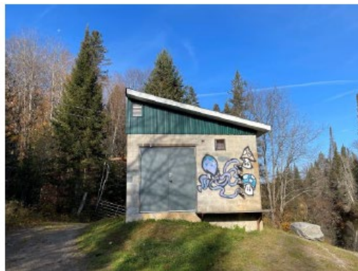
Photograph No. 1: Exterior view of the Nelson Pump Station building located at close to 220 Centre Street, Burk's Falls, ON.
