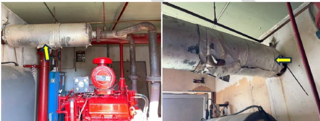
Photograph No. 2.1 and 2.2: View of asbestos-containing insulation associated with the muffler of the generator exhaust system within the subject building.
