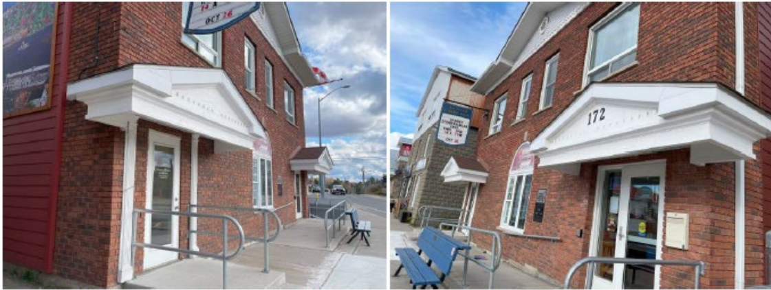
Photograph No. 1.1 and 1.2: Exterior view of the Municipal Office Theatre building located at 172 Ontario Street, Burk's Falls, ON.
