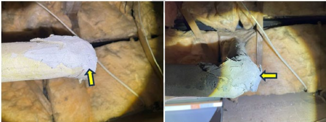
Photograph No. 2.1 and 2.2: View of asbestos-containing paring cement was identified on pipe fitting within the west office on the 1st floor municipal office of the subject building.
