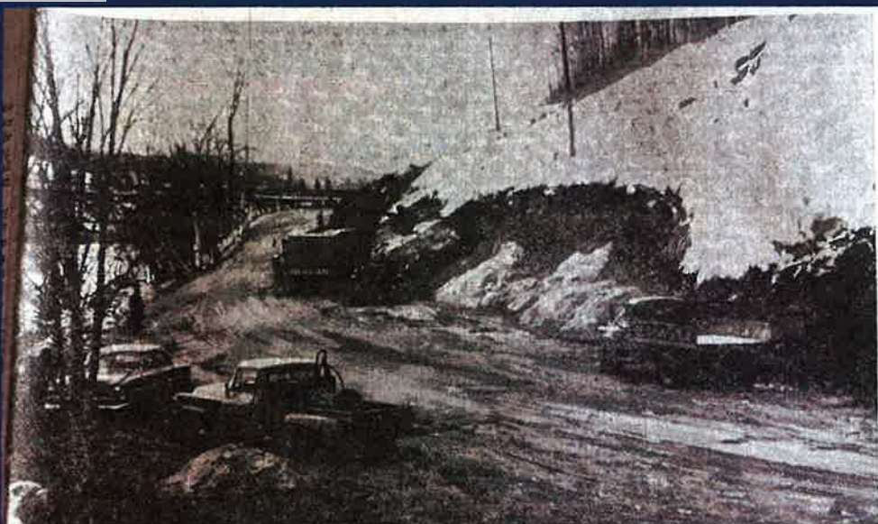
SCENE OF ACTIVITY — Shown here is the heavy equipment removing earth from the rock to be blasted in widening the Highway 520 in Burks Falls. Blasting operations have already started (Photo by Gough)
