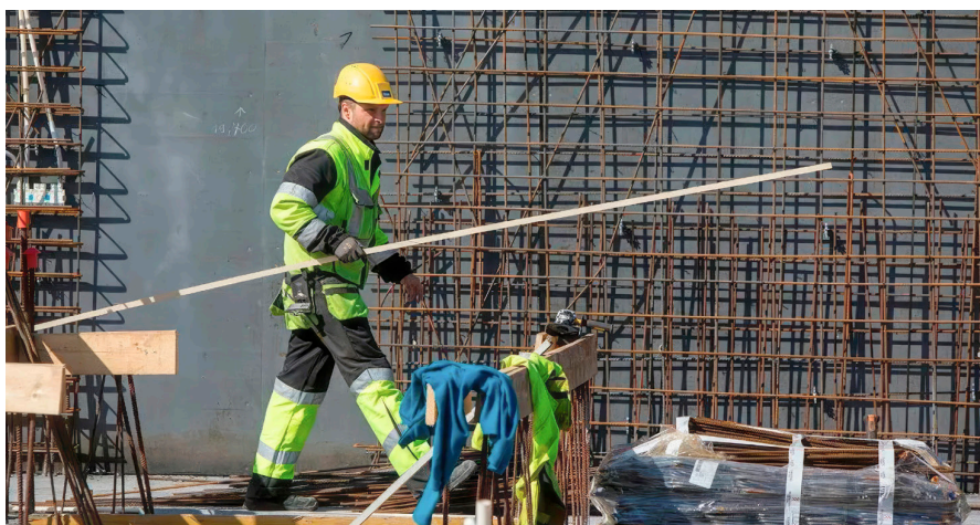
A construction worker on the job
