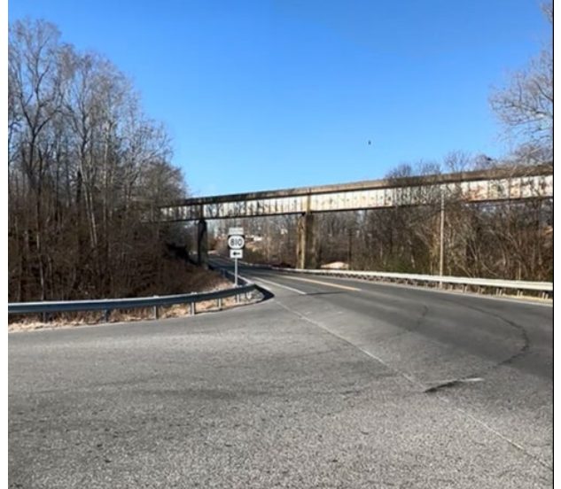
Figure 29: Signage limits sight distance for turning vehicles
