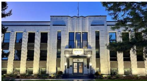
Washington County Courthouse - 256 E. Court Street (NRHP Ref# 87001602)
