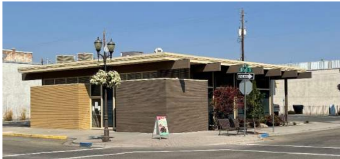
Former First Security Bank - 407 State Street
