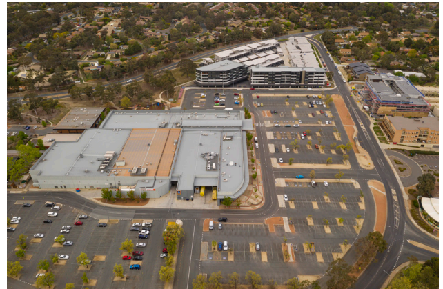
Carparks can create barriers to accessing local shops. Image credits: iStock.com; ai_yoshi and Steven Tritton
