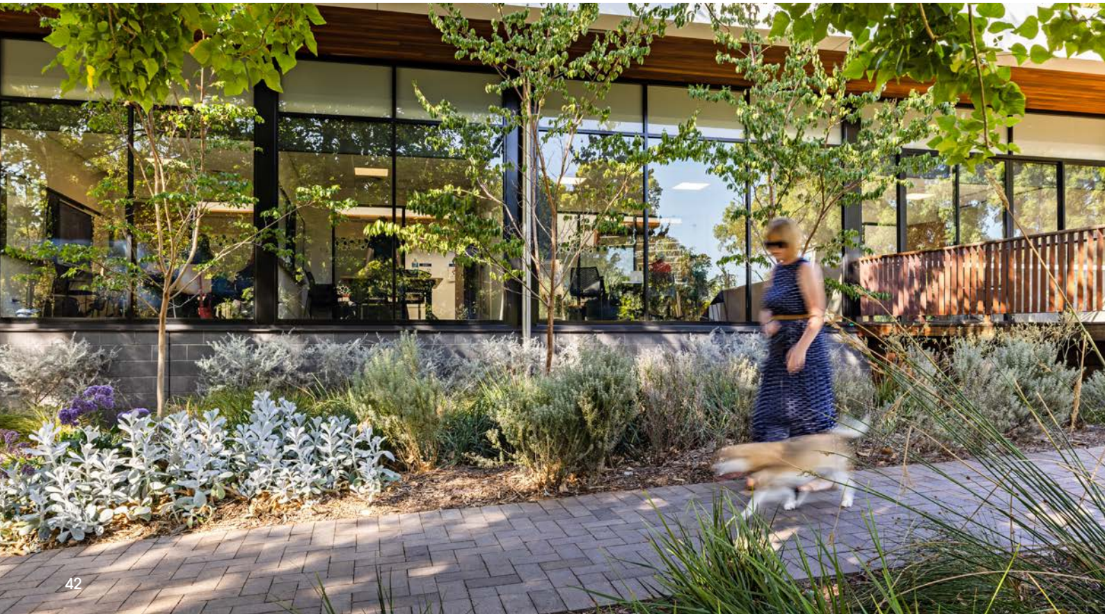
Mitcham Library and Brown Hill Creek, Mitcham. Terraced deck connects the library to the restored natural creek and surrounding public open space, creating a welcoming civic space for community gatherings, nature play and everyday recreation. Photo: supplied by ASPECT Studios, photography by Sweet Lime Photo .
