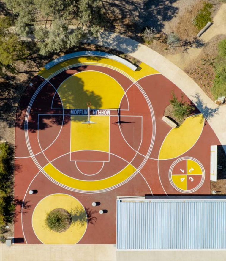
Mofflin Reserve Playground, Elizabeth Vale. Sport facilities integrated within Mofflin Reserve provide spaces for physical activity, supporting active lifestyles and social connection. Photo: supplied by LANDSKÅP, photography by Jack Fenby .
