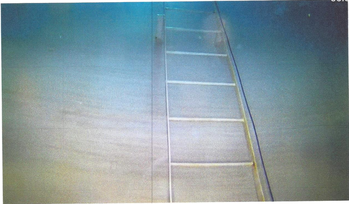
12.) Primary Interior Access Ladder
