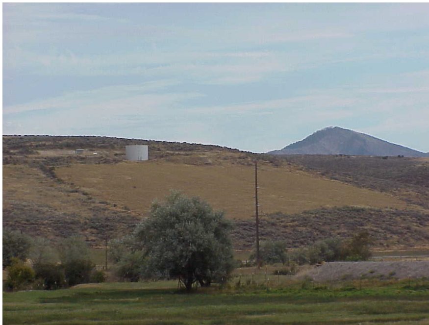
Figure 1-4 300,000 Gallon Water Tank
