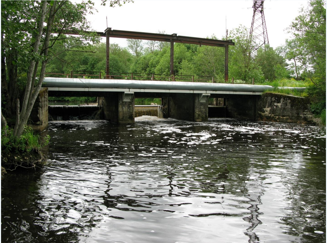
Photo 11. View to the Püssi dam on r. Purtse.
