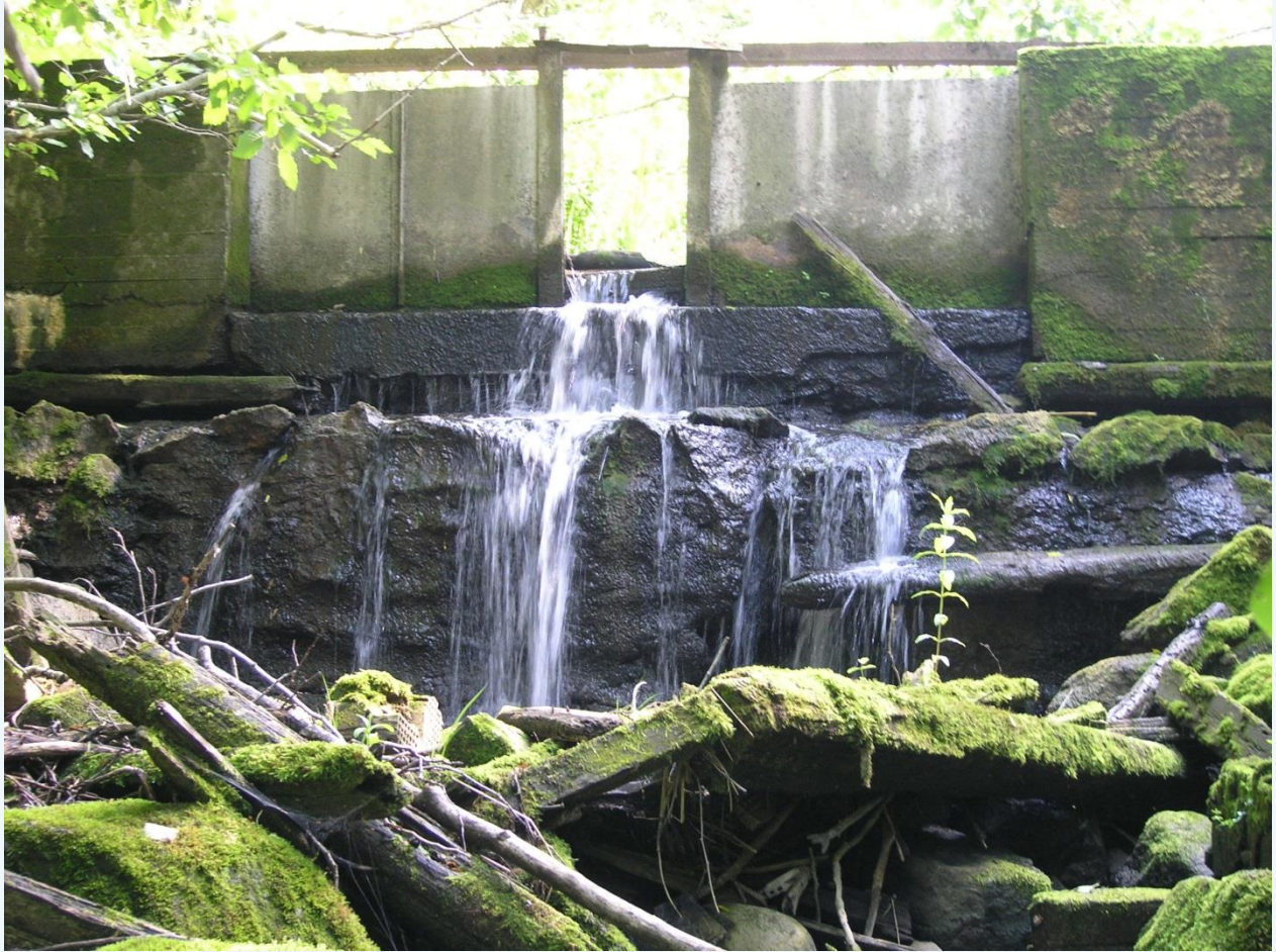
Photo 8. The 1.9 m high dam on Udria brook prevents access to about 75% of the potential sea trout spawning areas.
