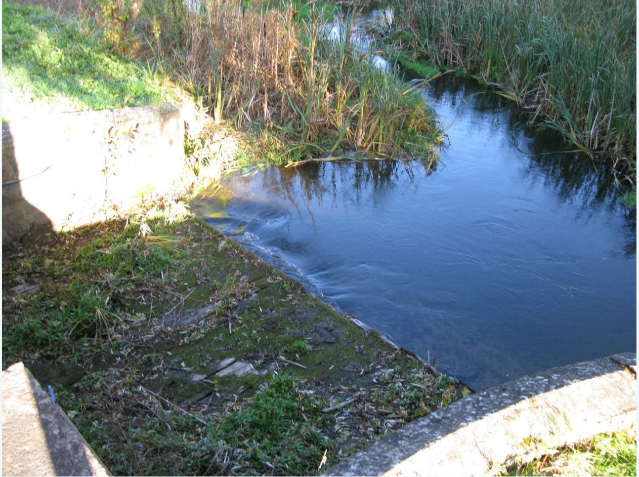
Photo 10. View to the upper part of the Undla dam.
