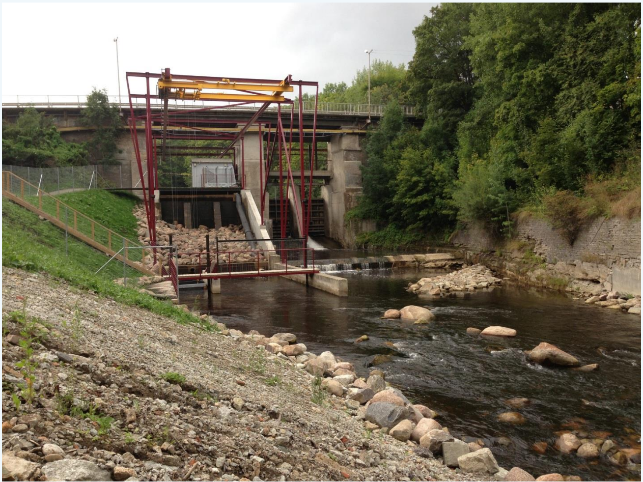
Photo 3. Kunda second Hydro hydroelectric power station has a fish lift that is considered not to provide sufficient passage.
