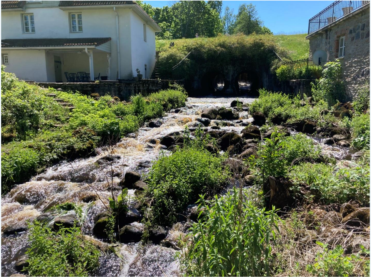
Photo 14. The two culverts below the regulator are in a steep angle and somewhat difficult to pass.
