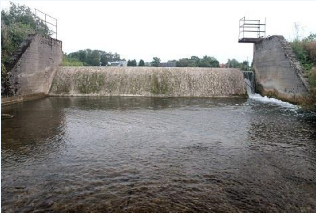
Foto 12. Presently the 1.6 m Ruila dam is the first definite migration obstacle for fish (G. Lauringson, 29.07.2013).
