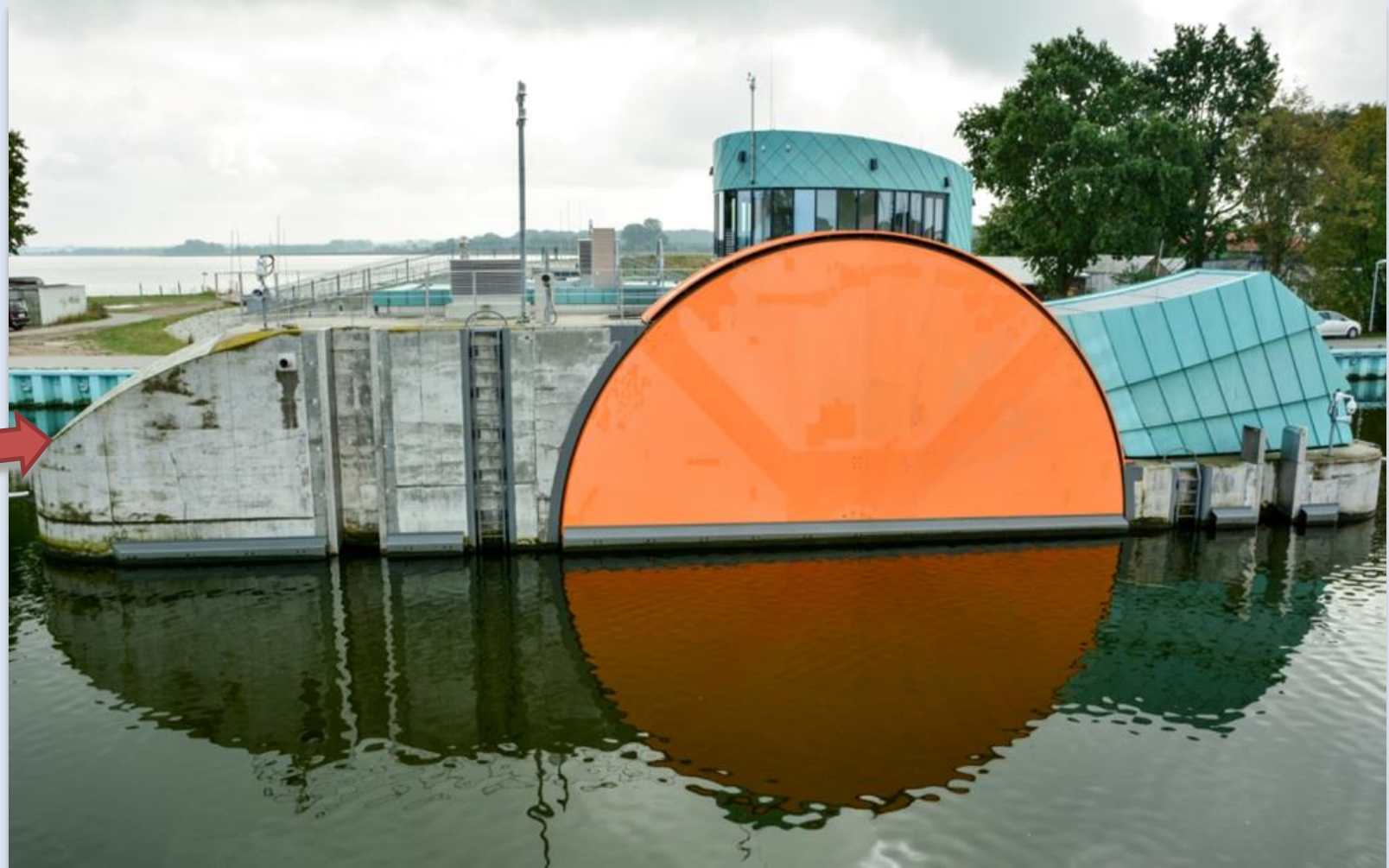
Flood gate (lock) in the river. Greifswald, Germany
