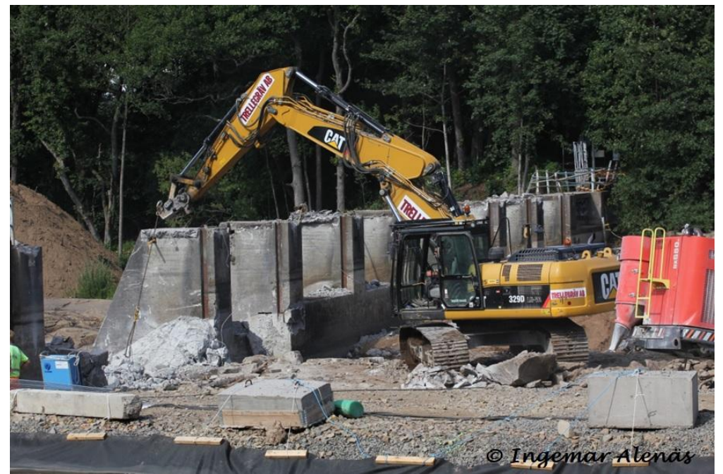
Removal of the Herting dam Falkenberg, partly funded by SSS NC's Good Environmental Choice
